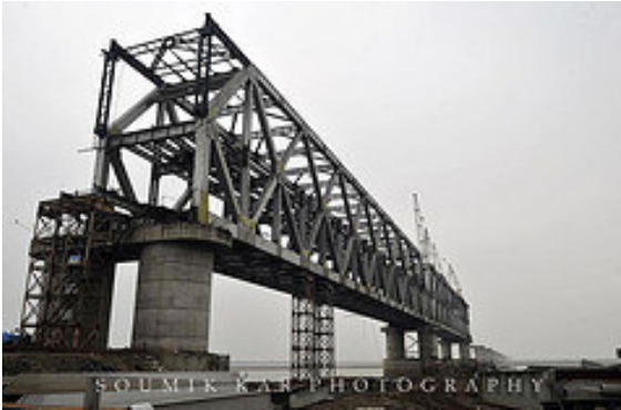
Figure 3: Ganga rail cum road bridge under construction
