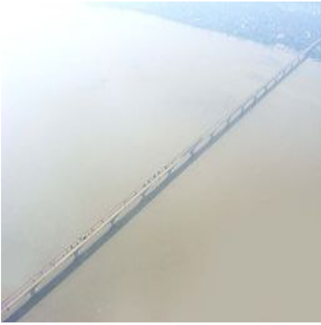
Figure 1 : TOP VIEW OF THE ROAD BRIDGE
