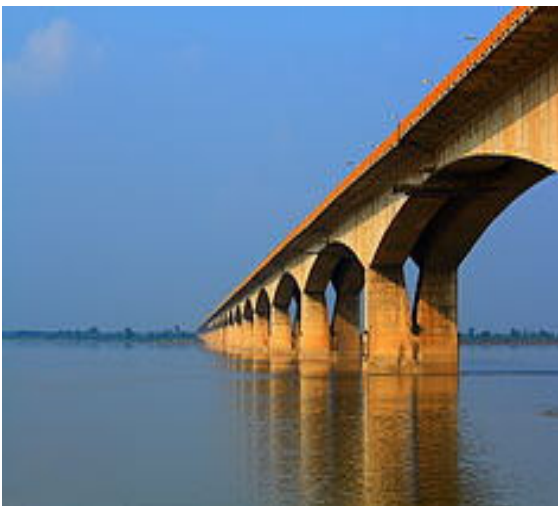
Figure 2: Cantilever structure of the bridge
